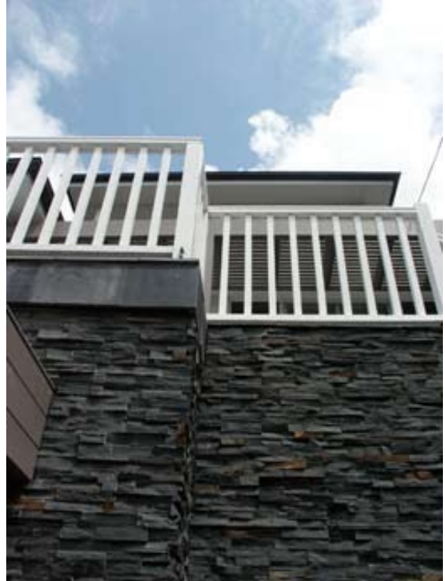
cladding to front of house
