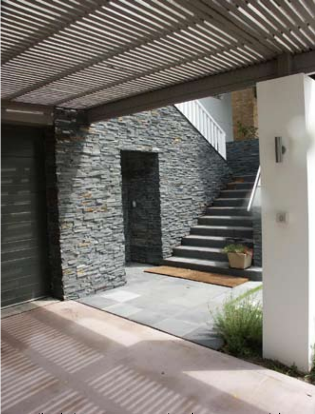
connection between new carport and new access stair
