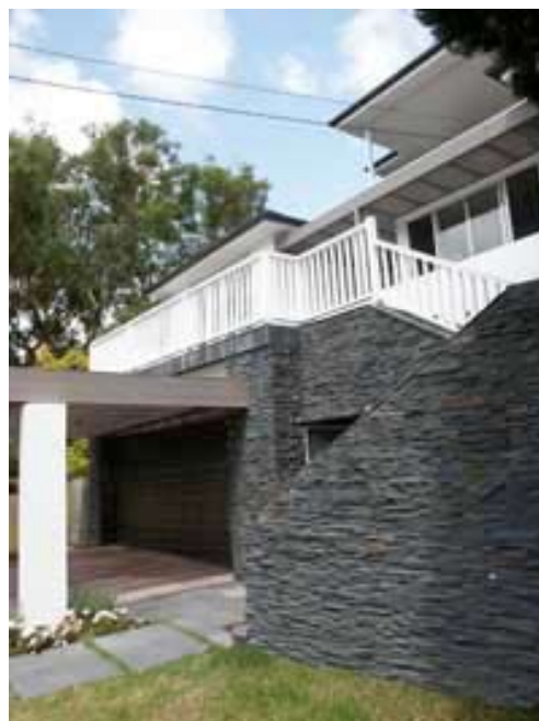
complete face lift to front of the house
